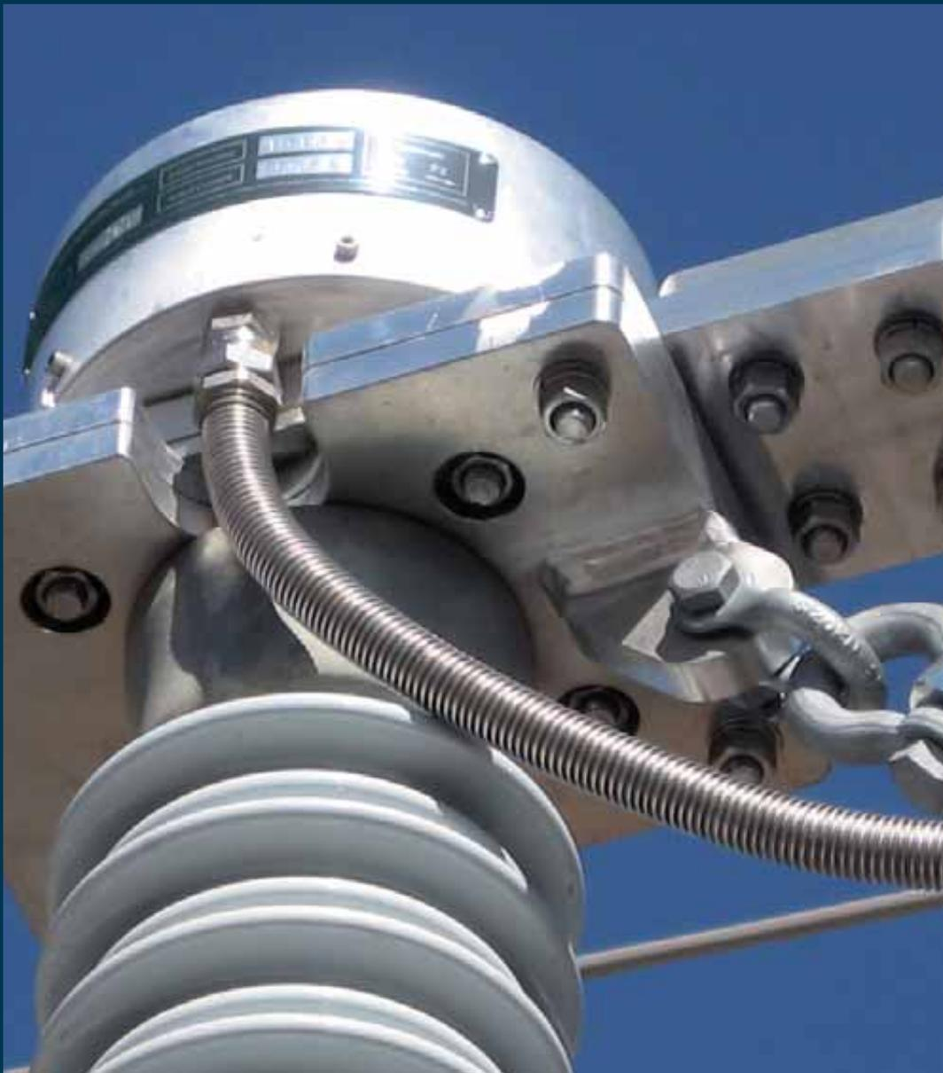
› Optical current transformer SDO OCT.
